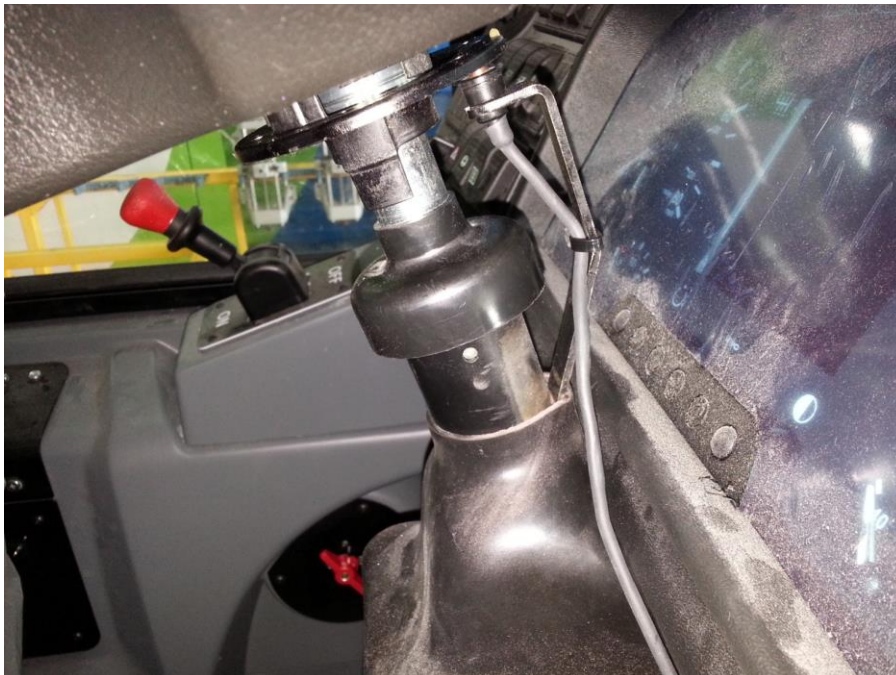
Figure 1: New bracket installed – welding complete, finish painting yet to be done.
