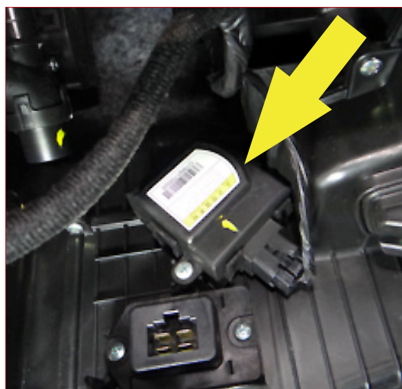
Fig. 2. Cluster ionizer location (by blower motor)
