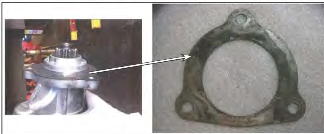
Figure 5 - Removal of Shim
