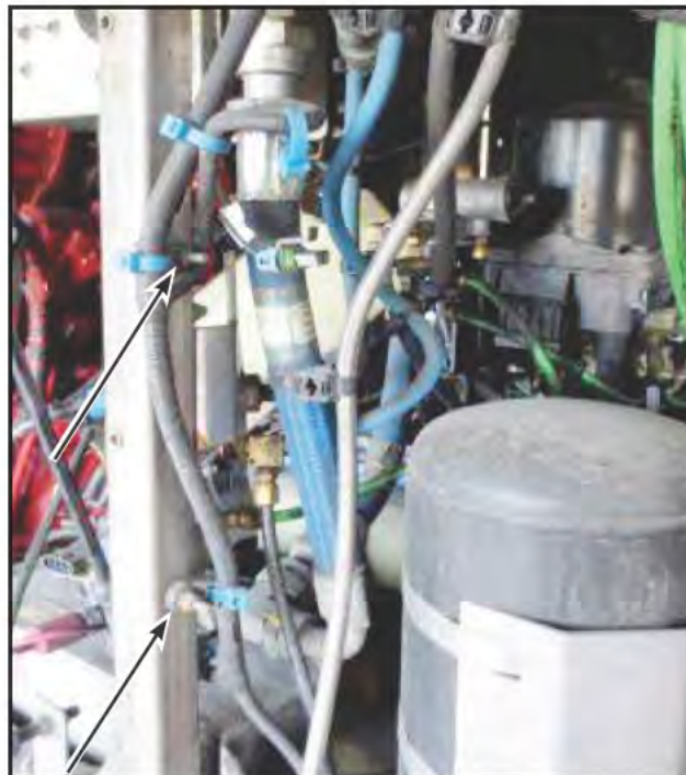
Figure 9 - Remove Electrical Harness from Structure
