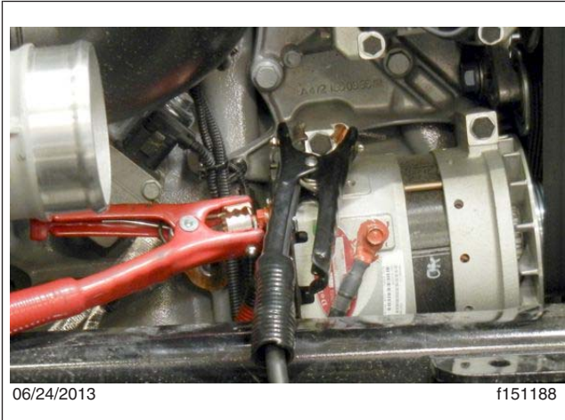
Fig. 7, For EPA10 and EPA04 engines, the starter path can be checked by loading the circuit at the alternator.
