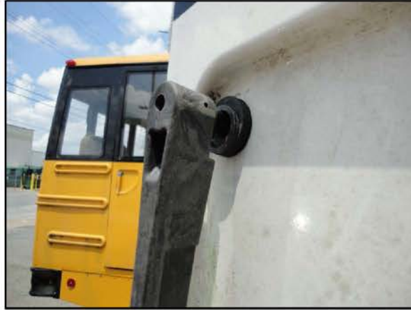
Figure 11, Position of Newly Installed Exterior Handle
