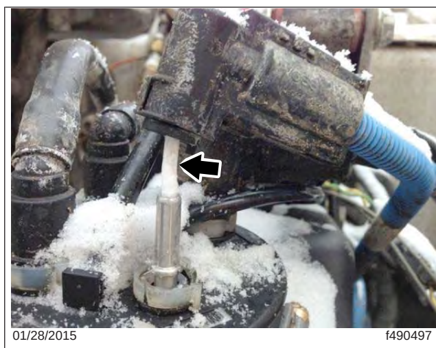
Fig. 1, Ice Expansion at the DEF Line Fitting
