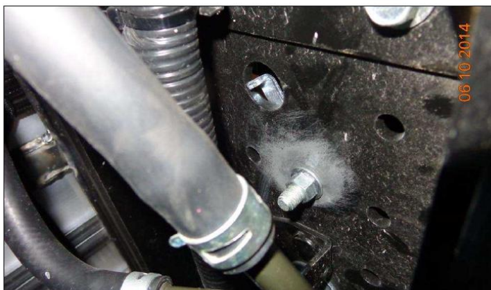
Cleansed starter ground at frame rail.
