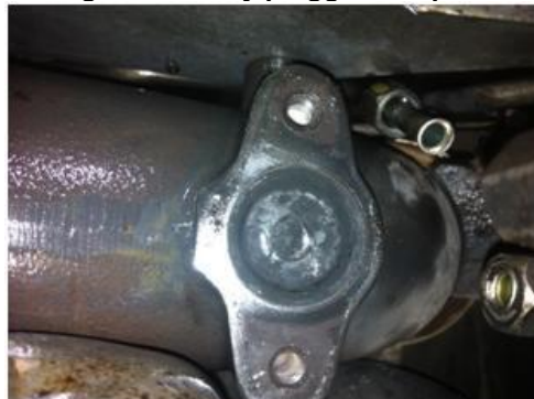
Figure 3 – Fully plugged AFI port
