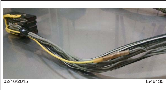
Fig. 5, Splicing the Wires
