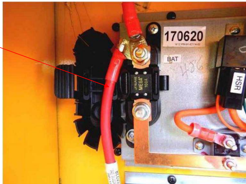
Figure 1, Incorrect Routing
