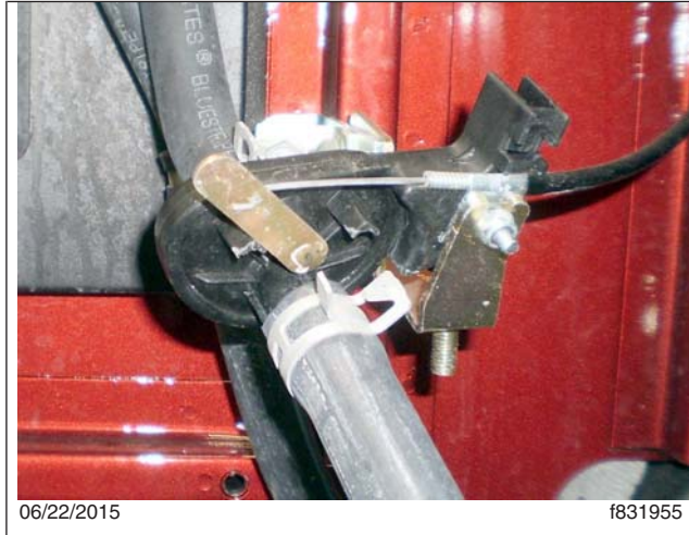
Fig. 13, Water-Valve Arm Resting on the Stop
