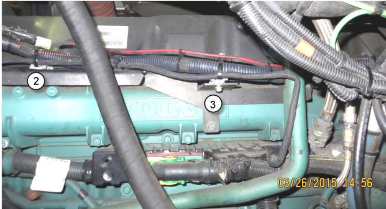
FIGURE 15: POWER CABLE ATTACHED TO #2, #3 DOUBLE-TIE MOUNT AND PROPER NYLON TIES INSTALLATION
