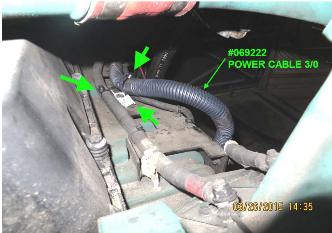
FIGURE 13: POWER CABLE ATTACHED TO #2 DOUBLE-TIE MOUNT AND PROPER NYLON TIES INSTALLATION
