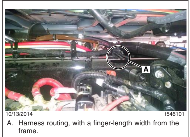
Fig. 2, Aftertreatment Harness Routed Along the Frame
