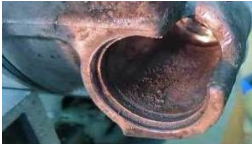
Figure 10. Corrosion in the N280 valve bore.
