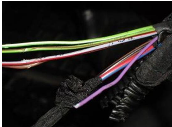
Figure 2. Wire harness under driver's side headlight.
