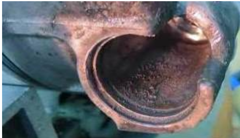
Figure 10. Corrosion in the N280 valve bore.
