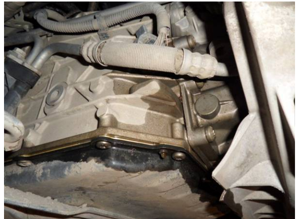
Figure 3. Leak between gearbox housing and intermediate housing.
