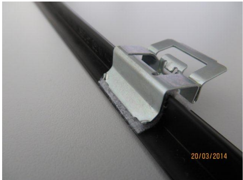
Figure 4: Retaining clip isolated with the fleece tape.
