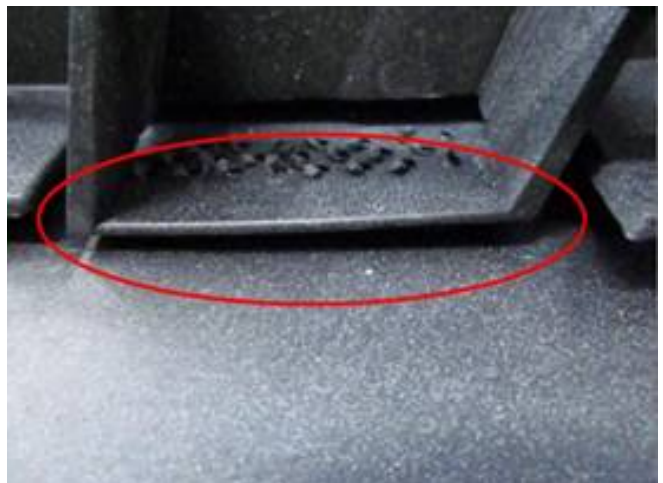
Figure 4. Loose mounting bracket.
