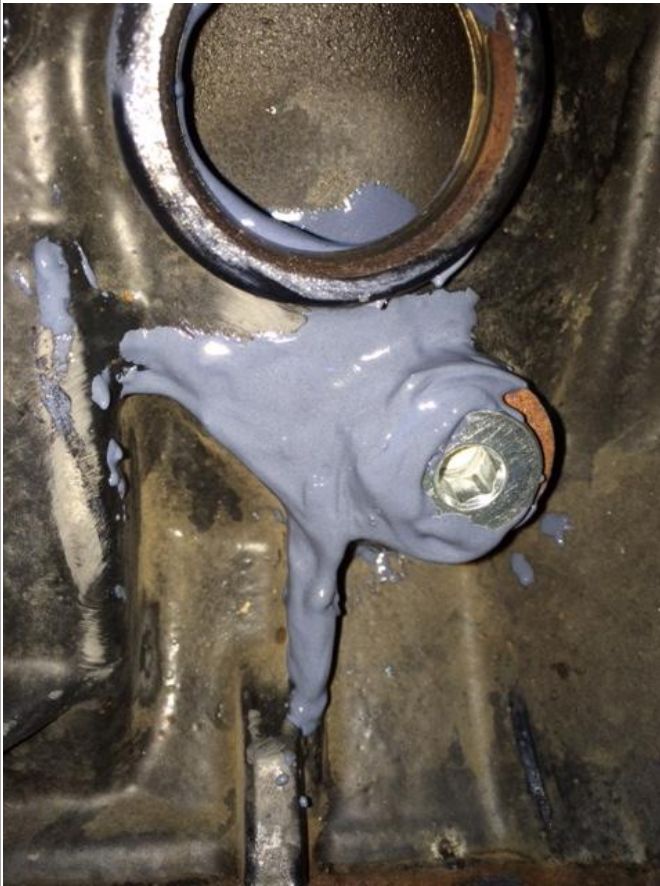
Figure 28: Use a Heat gun to Cure the Epoxy
