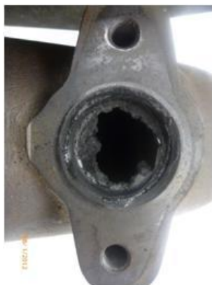
Figure 2 – Partially plugged AFI port
