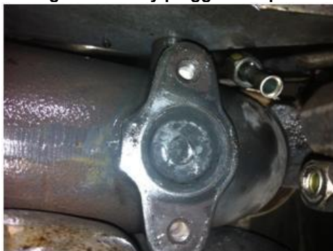
Figure 3 – Fully plugged AFI port
