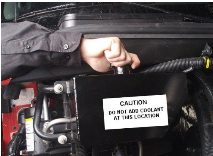
Figure 1 - Pressure Cap Installed on Expansion Tank
