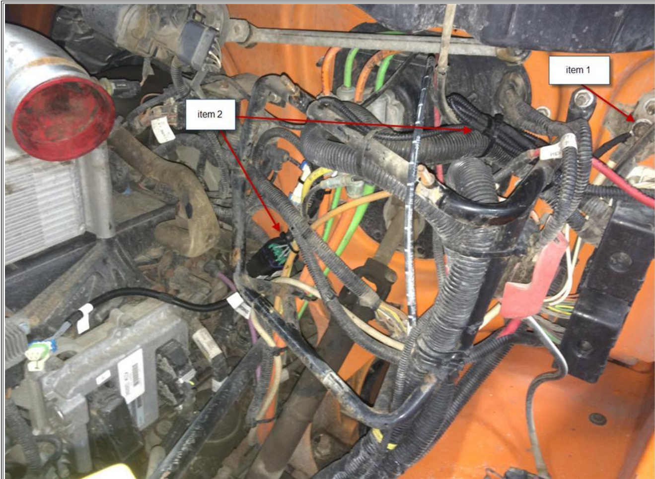
Figure 3: Suggested Harness Routing for Big bore engines (15" housing)
