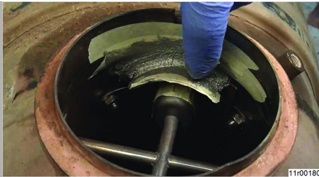
Figure 11: Applying High Temp Sealant to Water Shield
