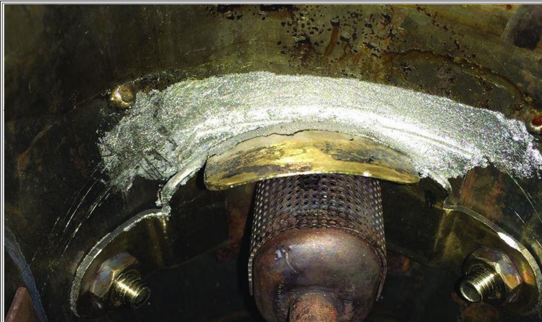
Figure 12: Masking Tape Removed from Water Shield
