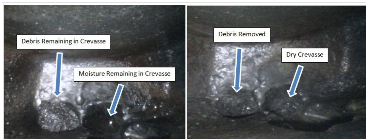
Figure 19: (LEFT) Coolant Galley with Moisture and Missed Debris (RIGHT) Coolant Galley After Cleaning and Drying
