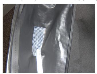
2. Apply a fiberglass mesh reinforcement tape to the topside of the hole. Ensure that the tape extends 25 mm (1.0 in) all around the hole.
