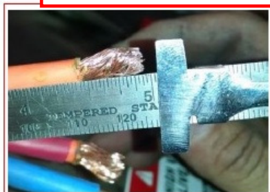
Measure exposed wire end after Repair for installation
