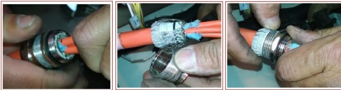
Repositioning the cable in the sealed cable gland assembly.
