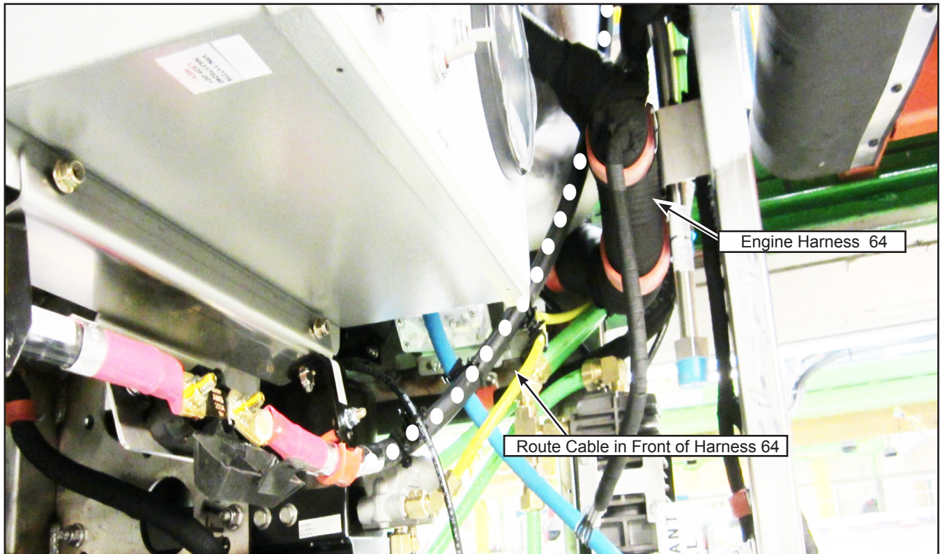
Figure 4 - Routing and Clamping of Right Power Cable
