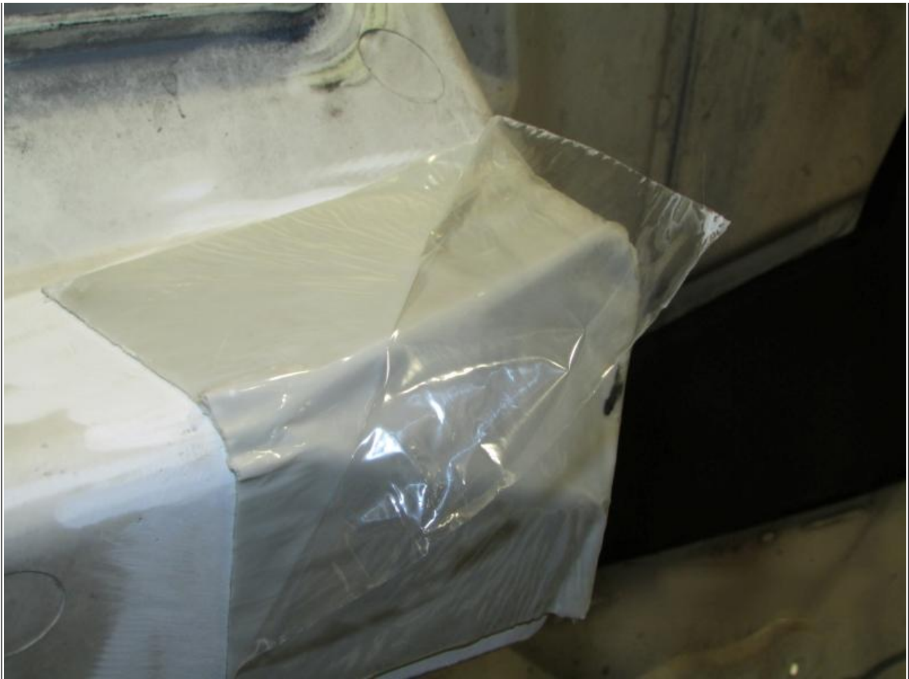
Figure 9: Patch placed and formed.
