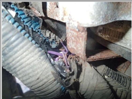
Figure #2: Harness chafing(incorrectly routed)
