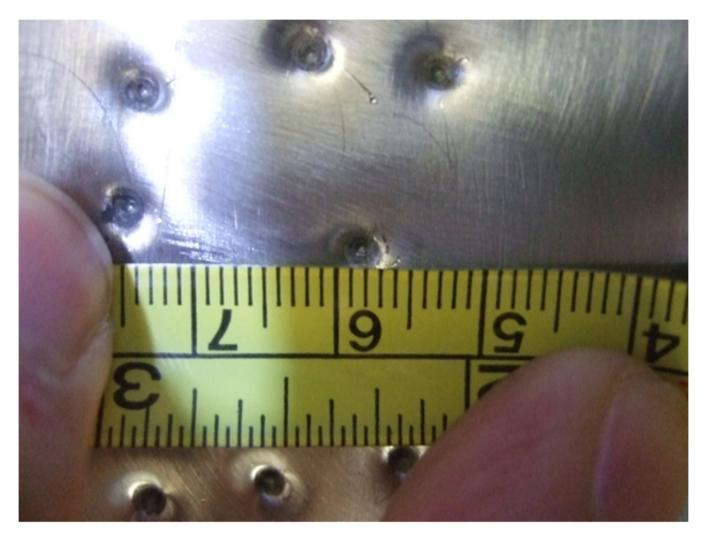
Do not be concerned if the gap between the outer and middle sheet metal increased as a result of punching. No attempt should be made to flatten this area. Leave it raised.
