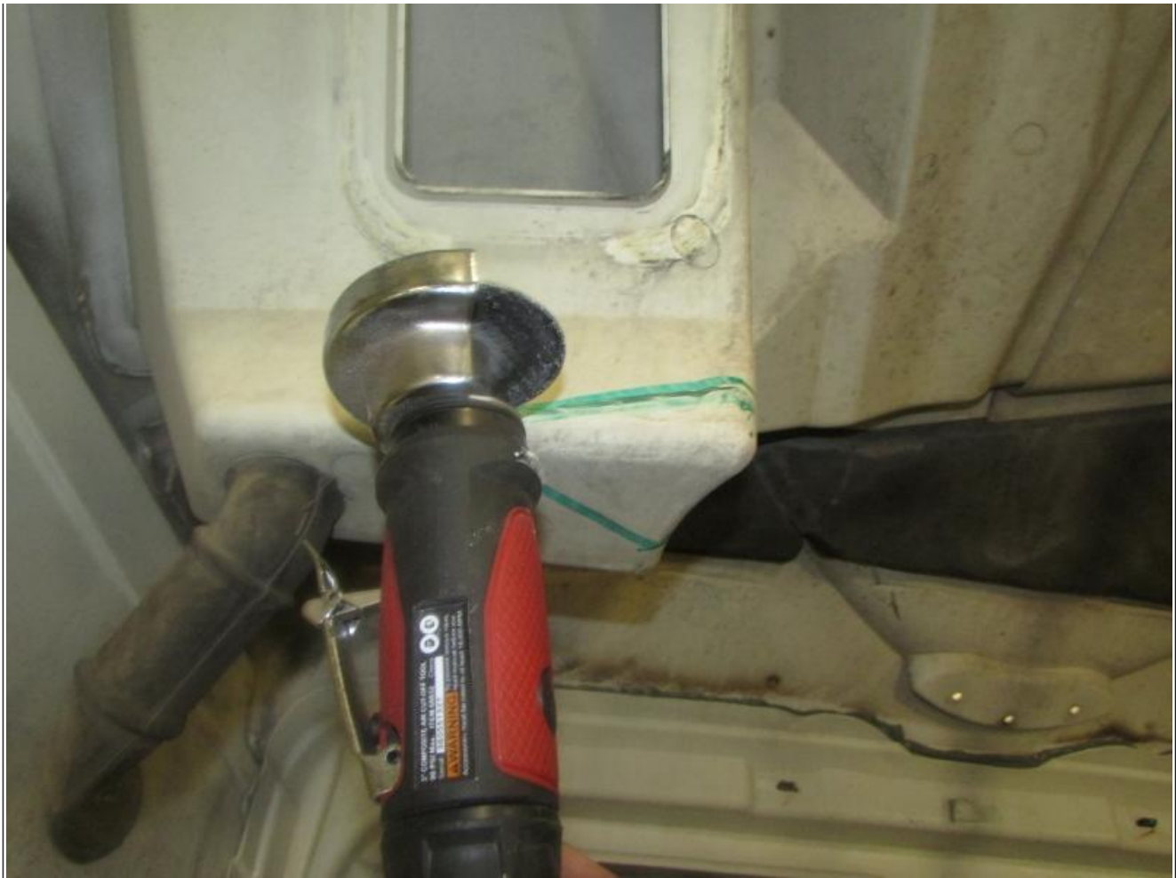
Figure 7: Die grinder material removal.
