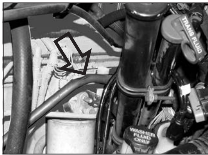
Damaged discharge line shown.
