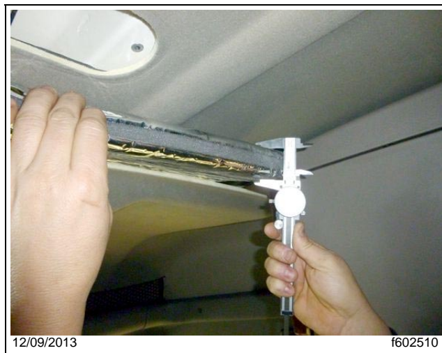
Fig. 3, Measuring Cab Roof Insulation Thickness
