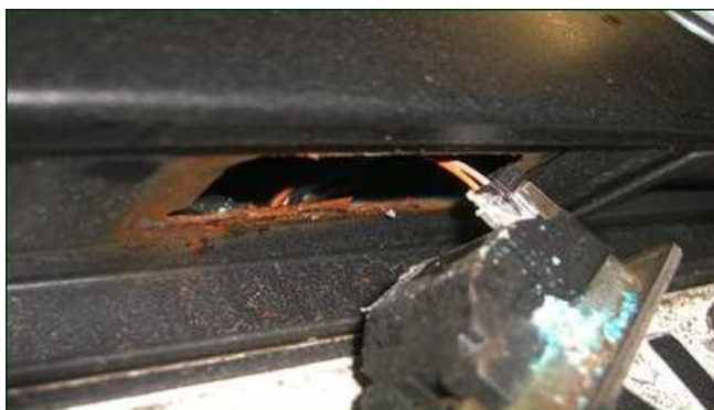
Figure 2: corrosion on opening for the number plate light - example AJ5, clipped installation
