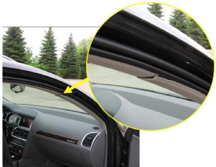
Figure 5. Loose A pillar trim.
