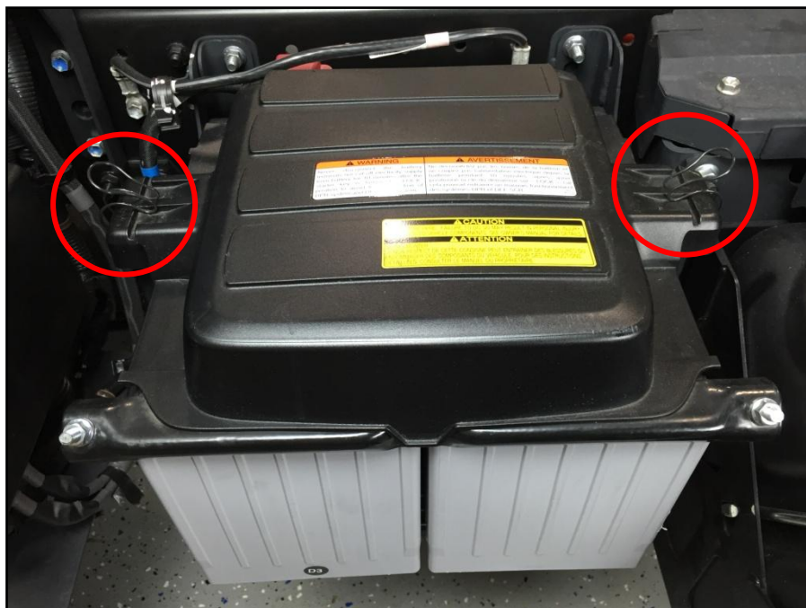
12 Volt Batteries Cover and Spring Clips
