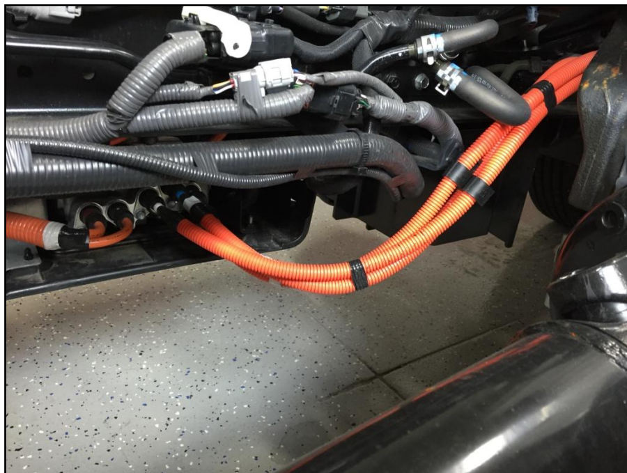
Orange Cables That Carry High Voltage Alternating Current (AC)
