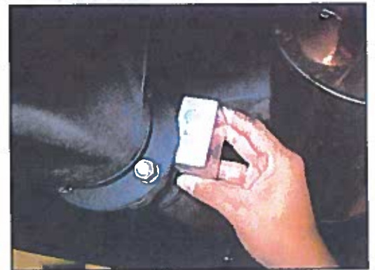
Figure 13. INCORRECT Placement of Protractor
