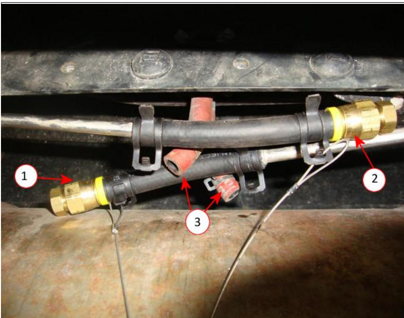
Photo 3 - EGDP Plugs and Hoses Installed on Steel EGDP Tubes EGDP Plug EGDP Plug Original hoses to EGDP Sensor disconnected
