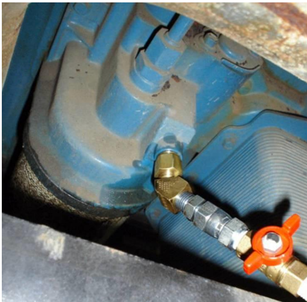
Figure 5: Oil Supply Feed Line connected to Oil Filter Header
