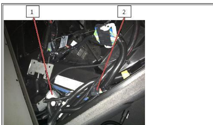
Figure 1: Control Center Harness.
