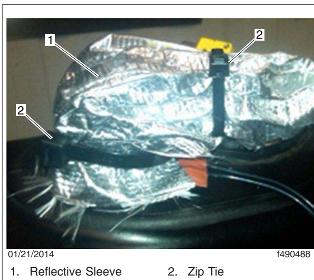
Fig. 4, Installing the Reflective Sleeve
