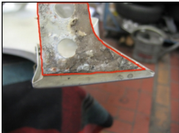
Figure 2 - fender removed (corrosion on the contact surface of the fender)
