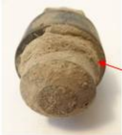
Clogged With Debris
