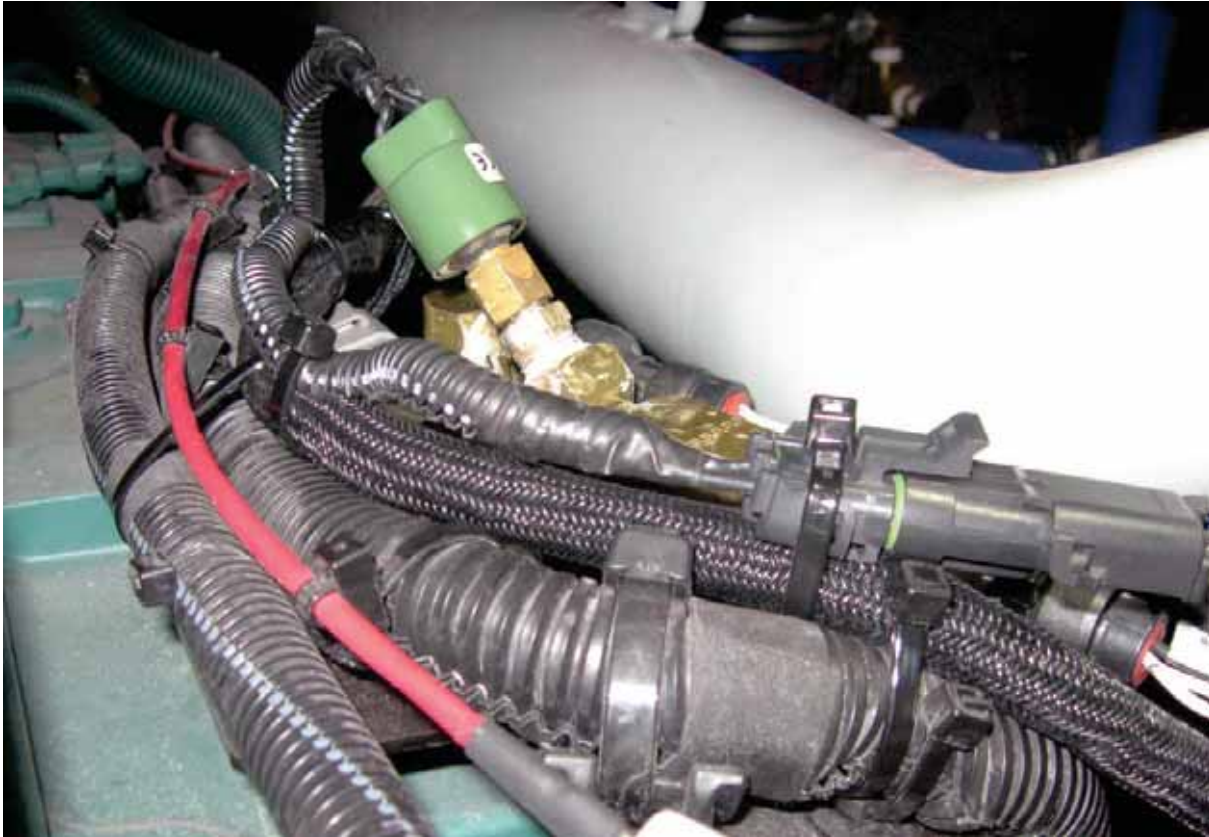
Figure 25 : SE29 view from rear.
