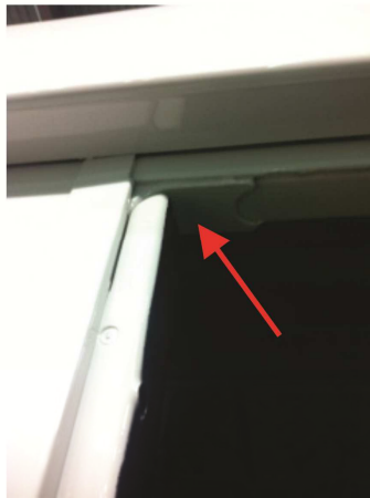
FIGURE 9 A: SHOWN COMPLETED VIEW OF CORNER GUSSET PLATES WELDED IN PLACE.
