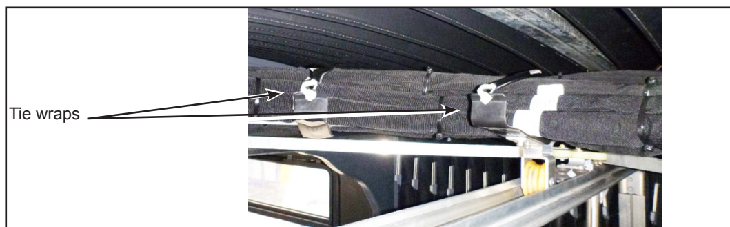
Figure 34 - Tie Wrap Installation
