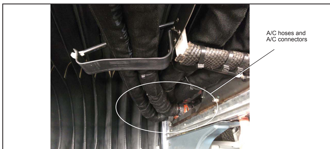
Figure 35 - No Contact Between Hoses and Surrounding Components
