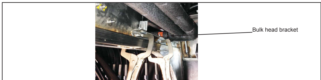
Figure 7 - Fixing the Bracket
