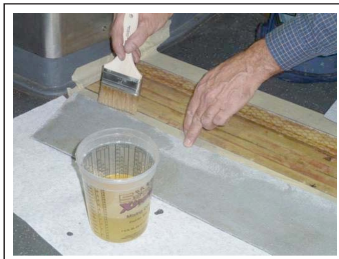
Figure 13 - Applying Adhesive on Floor Covering
