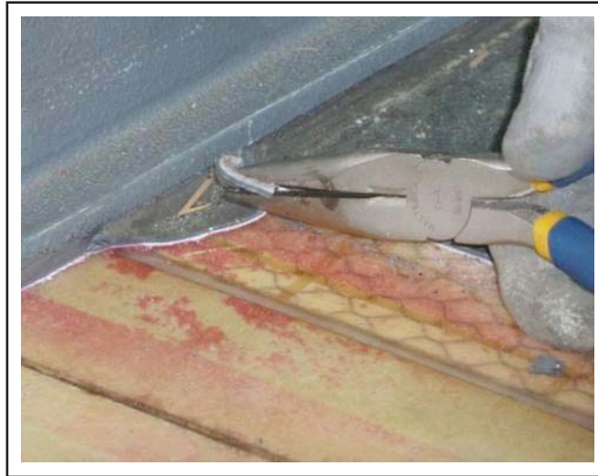
Figure 10 - Removal of Remaining End Sections
