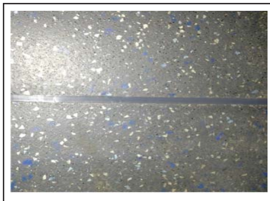
Figure 7 - Good Floor Seam
