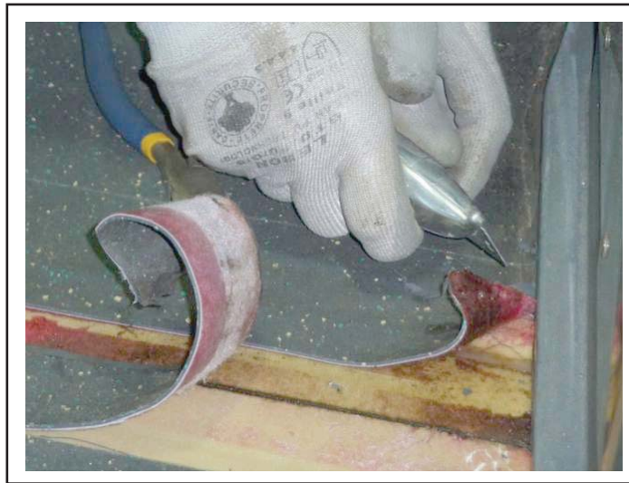
Figure 8 - Removal of Damaged Section
