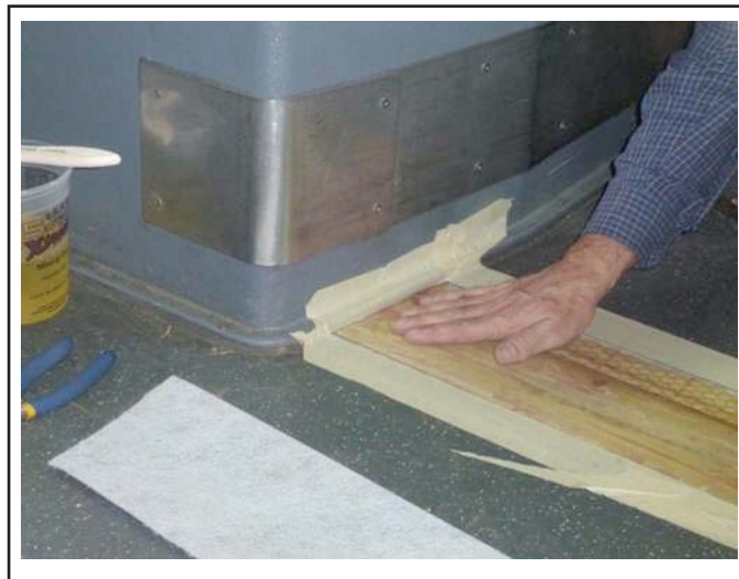
Figure 11 - Applying Masking Tape to Protect Surrounding Areas
