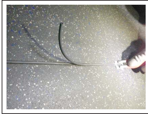
Figure 5 - Removal of Extra Material Using the Mozart Knife with the Attached Plate
