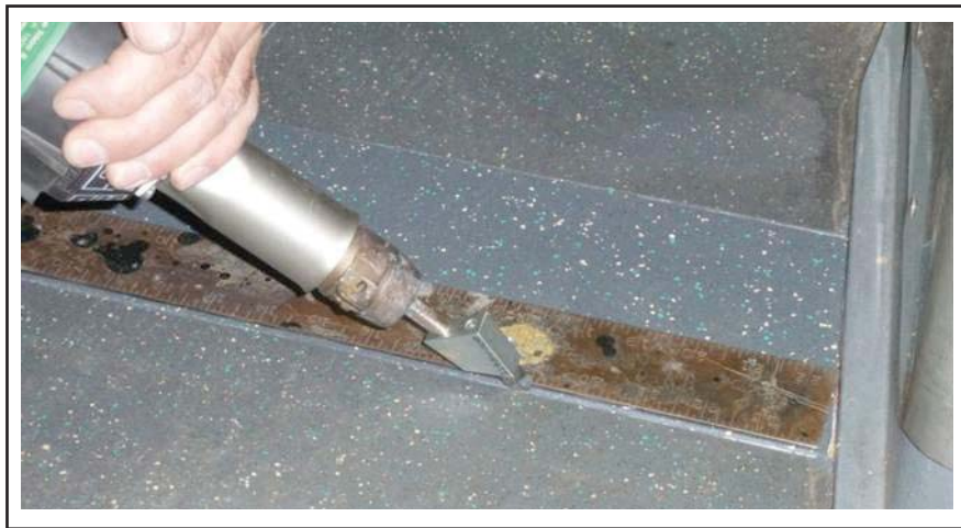
Figure 14 - Creating a Groove on Both Sides of New Bonded Piece of Floor Covering
