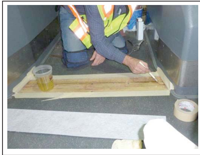
Figure 12 - Applying Adhesive on Floor
