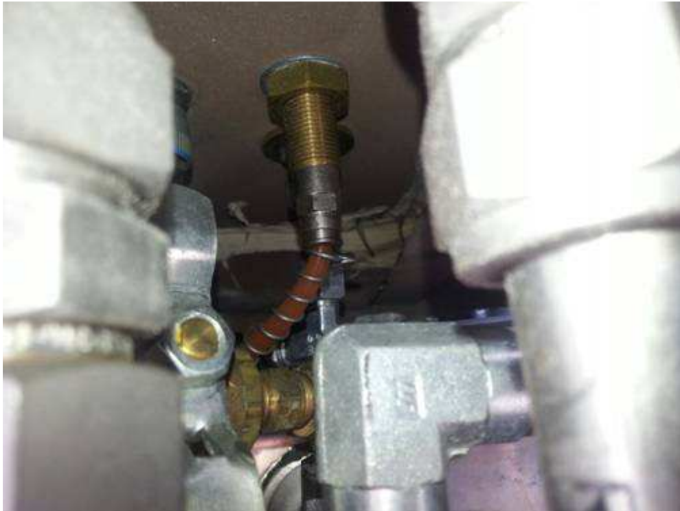
Figure 1: Bulkhead fitting and detector tube
